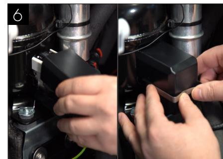
Install the new relay cover and secure with the securing clip, both found in your kit. Your relay replacement is now complete. Now move onto step 2.
